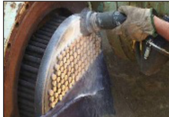
Surface preparation and tube protection
